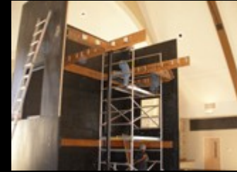
Structural steel and laminated beams installed to support the organ.
