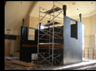
The swell box being erected.
