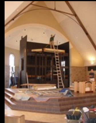
The organ structure is ready for casework and façade pipes.
