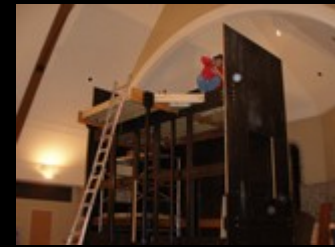
The second level and shade frames are going up.
