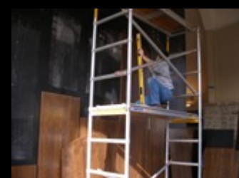
Finished panels being installed on the chapel side of the organ case.
